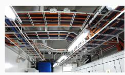
Interconnecting cables from the MEP to the DP, will consist of networking and control system cables. Routing these cables will have to be separate from any mains infrastructure.
